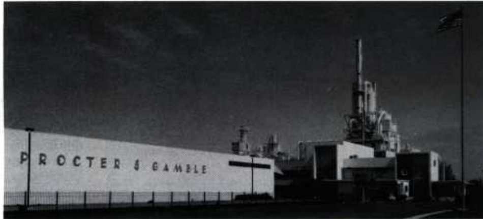
PROCTOR & GAMBLE MANUFACTURING CO. SACRAMENTO PLANT
